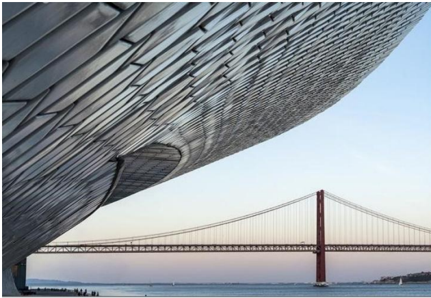
Curves and Cables 35
